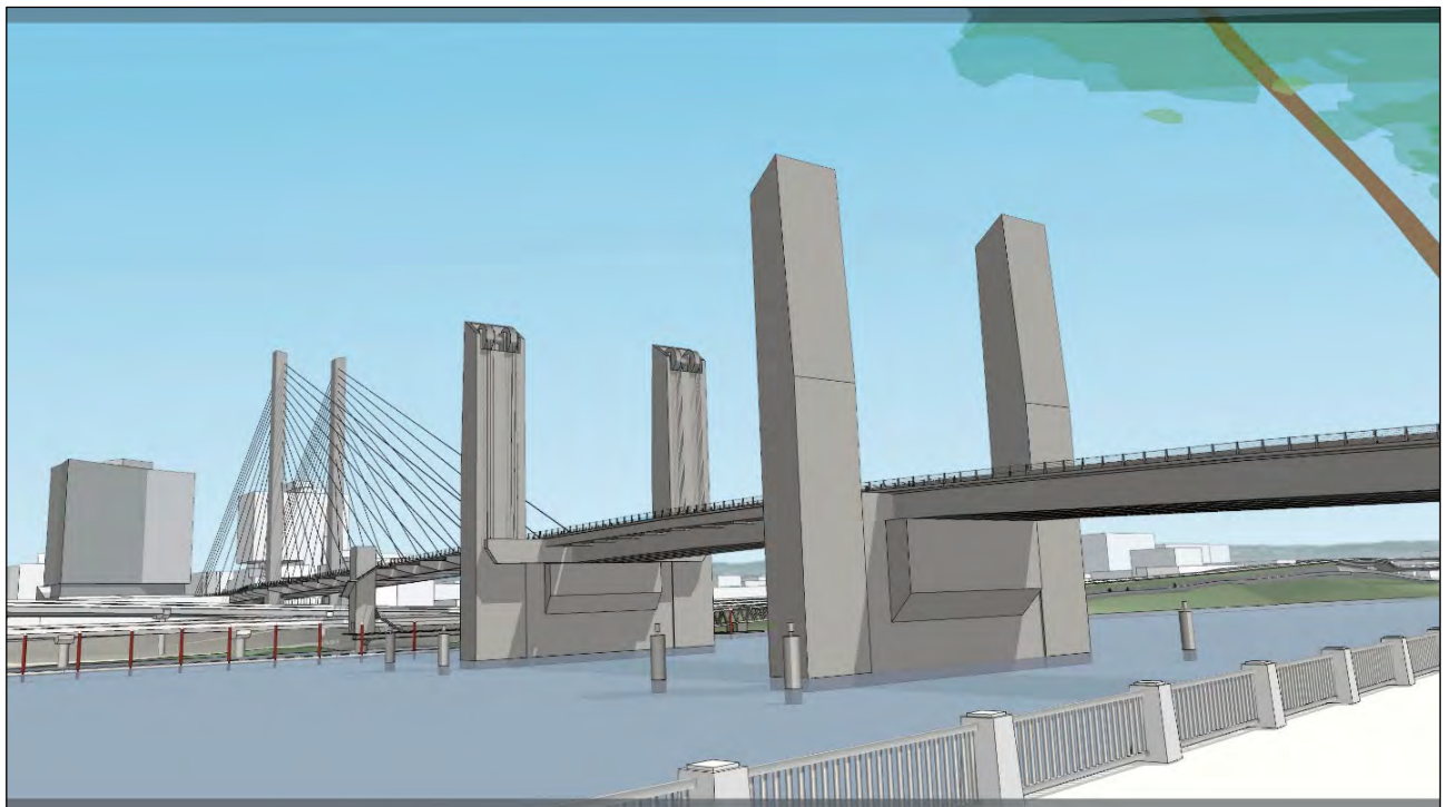
Figure 52: Span Combination 4 (girder west approach, vertical lift central span, cable supported east approach), artist's rendering, view looking southeast (Fat Pencil Studio, 2021).
