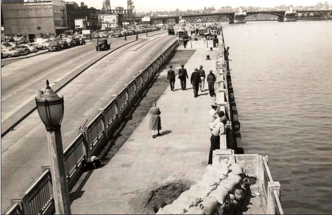
Figure 10. Harbor Wall reinforced in response to the June 1948 flood, looking north to the Burnside Bridge (Portland City Archives).
