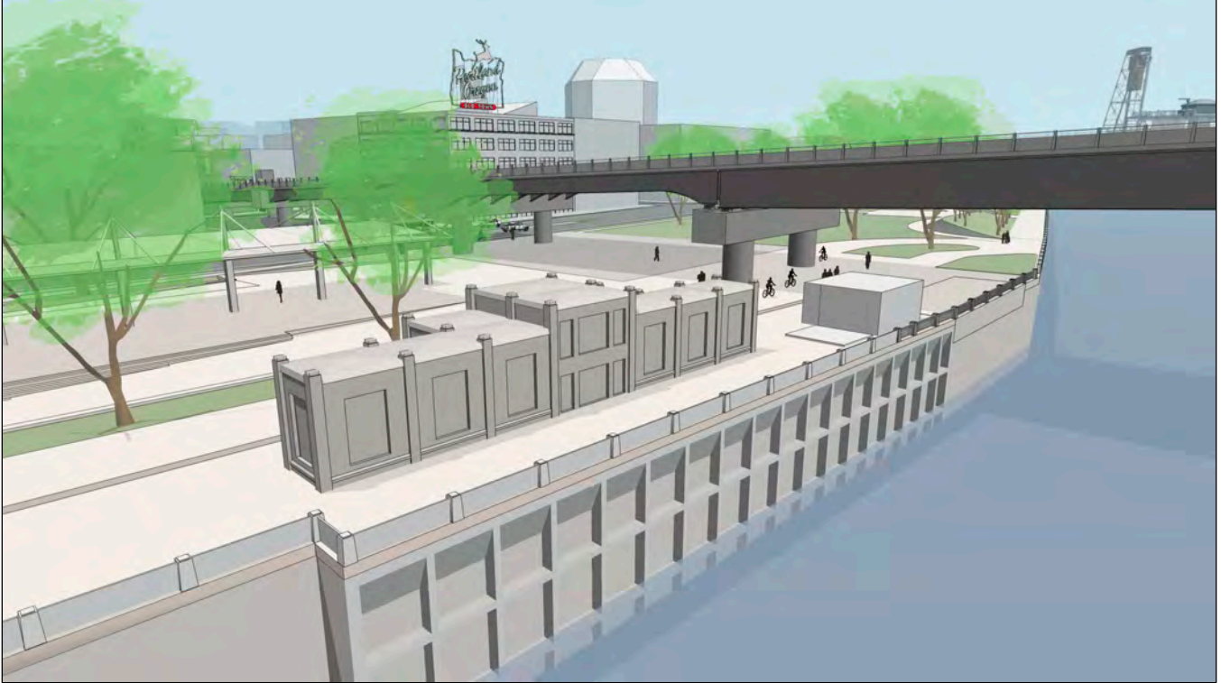
Figure 4. Portland Harbor Wall, artist's rendering (Fat Pencil Studio, 2021), oblique view looking northwest. This figure illustrates the condition of the Portland Harbor Wall after demolition of the existing Burnside Bridge, removal of Pier 1, and replacement of the west approach with a girder span.
