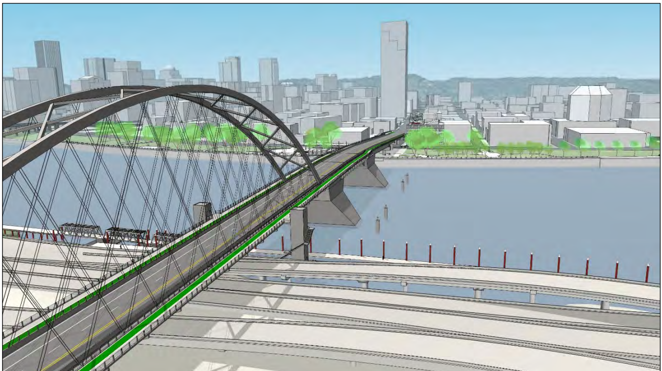
Figure 34: Span Combination 1 (girder west approach, bascule central span, tied arch east approach), artist's rendering, view looking southwest (Fat Pencil Studio, 2021).
