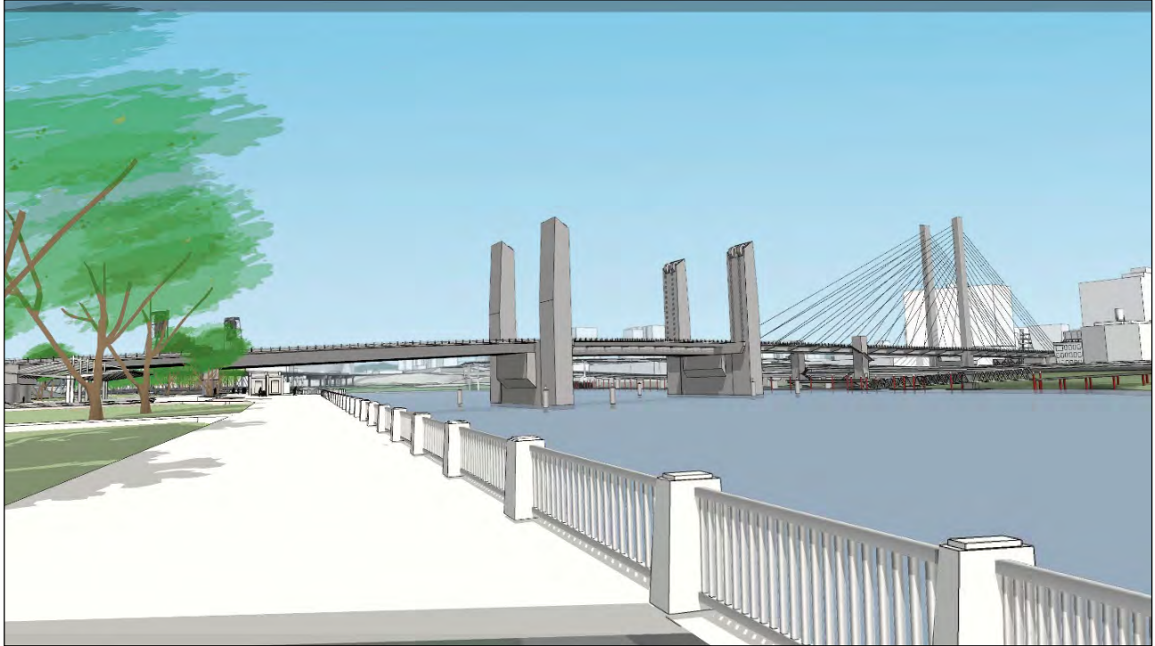
Figure 47: Span Combination 4 (girder west approach, vertical lift central span, cable supported east approach), artist's rendering, view looking southwest (Fat Pencil Studio, 2021).
