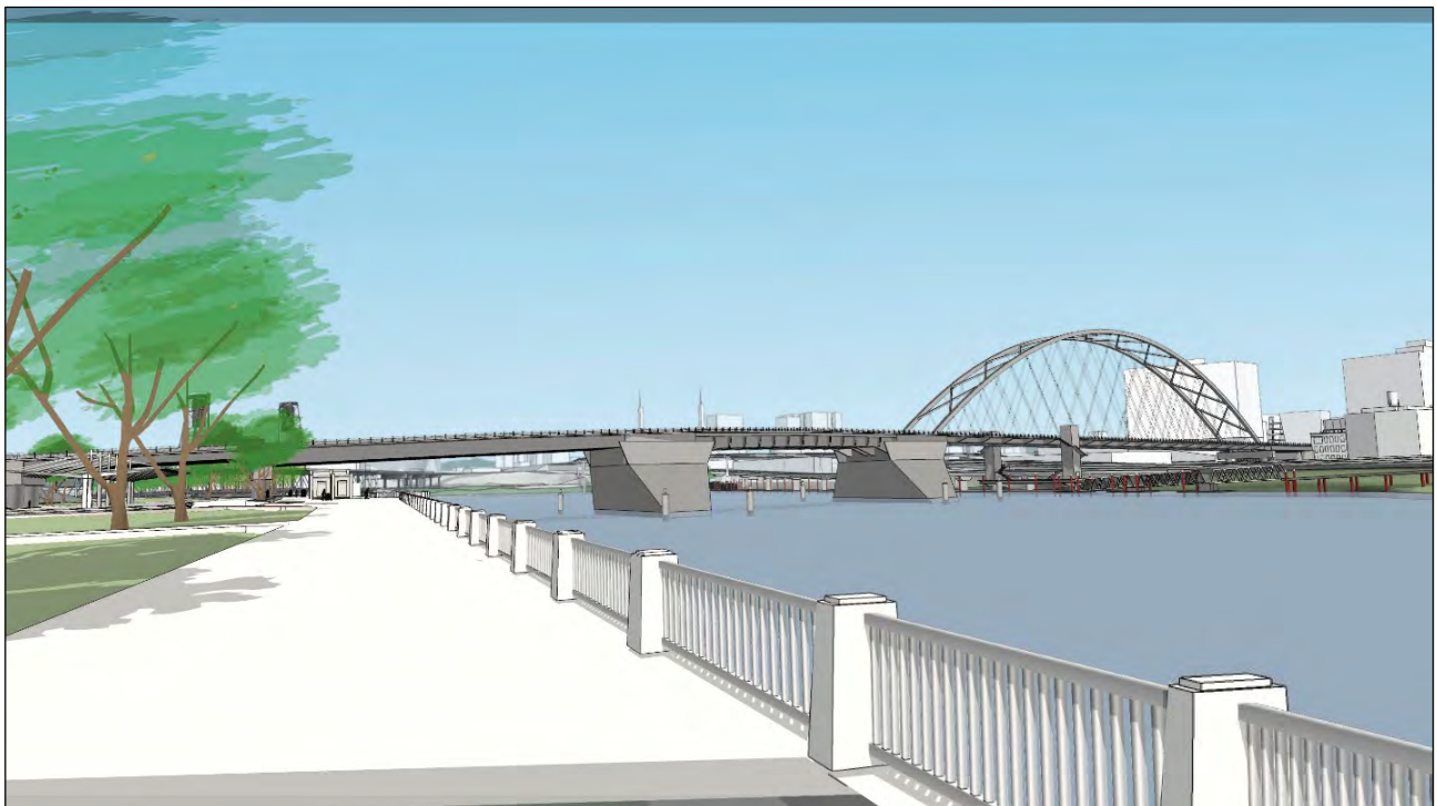
Figure 44: Span Combination 1 (girder west approach, bascule central span, tied arch east approach), artist's rendering, view looking north (Fat Pencil Studio, 2021).
