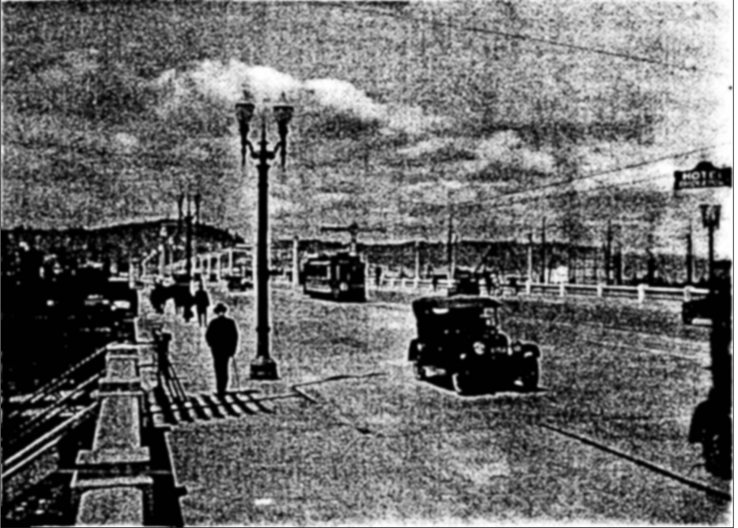
Figure 8: Photograph of Trolley Poles and Trolleys on the Burnside Bridge, circa 1926, courtesy Steve Dotterer. Note the section of guardrail to the west of the stair that is different than the concrete balustrade of the east approach. The Frigidaire Building was constructed immediately to the west of the stairway down to SE Third Avenue. (Historic American Engineering Record 1990).
