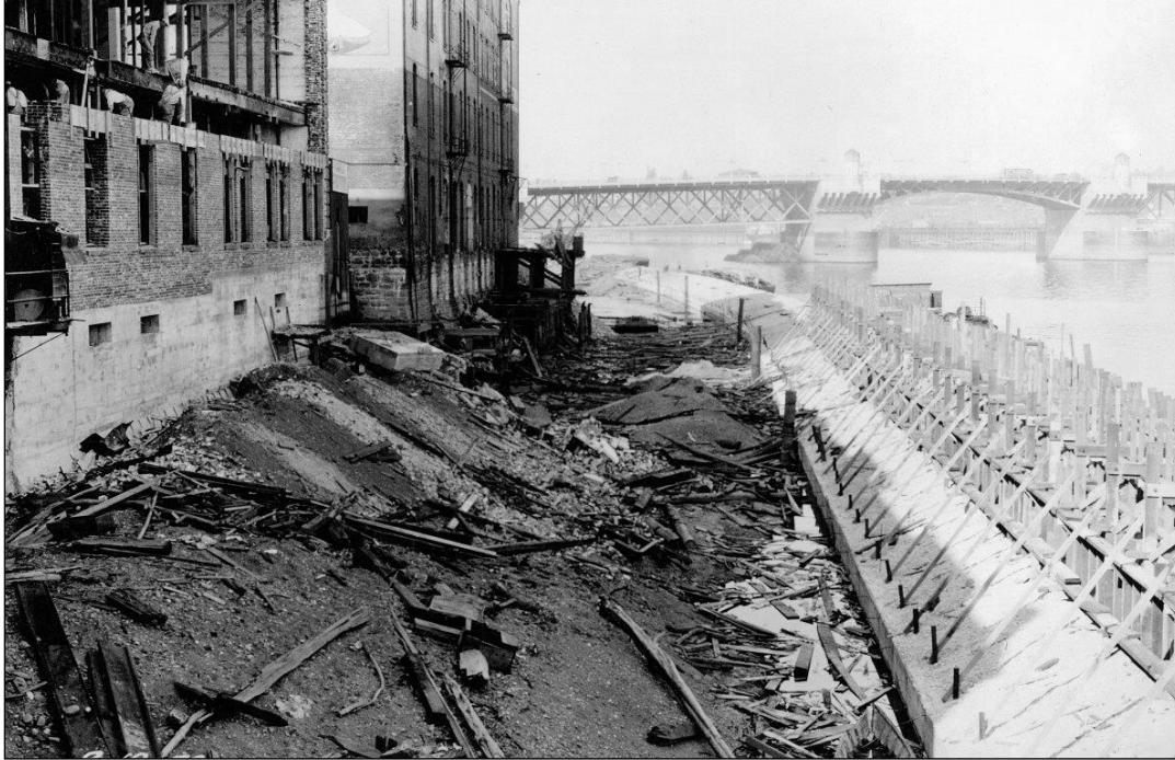
Figure 8. Harbor Wall under construction in 1929, looking north to the Burnside Bridge (Portland City Archives).
