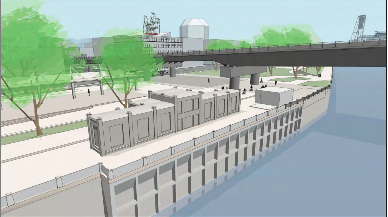
Figure 4. Ankeny Pumping Station, artist's rendering (Fat Pencil Studio, 2021), oblique view looking northwest. This figure illustrates the setting of the Pump Station after demolition of the existing Burnside Bridge, removal of Pier 1, and replacement of the west approach with a girder span.
