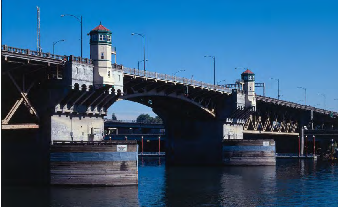
Figure 11: Detail of the operator's houses and drawspans of Burnside Bridge, looking northeast. Burnside Bridge, Spanning Willamette River at Burnside Street, Portland, Multnomah County, Oregon. Photos from Survey HAER OR-101 (Library of Congress).
