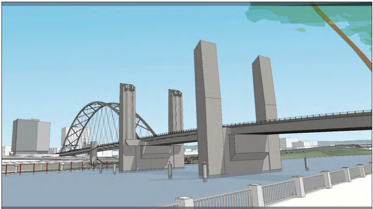
Figure 50: Span Combination 2 (girder west approach, vertical lift central span, tied arch east approach), artist's rendering, view looking southeast (Fat Pencil Studio, 2021).
